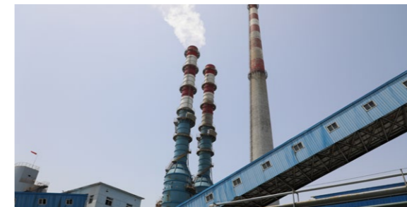
Desulphurization and Denitrification Facility
