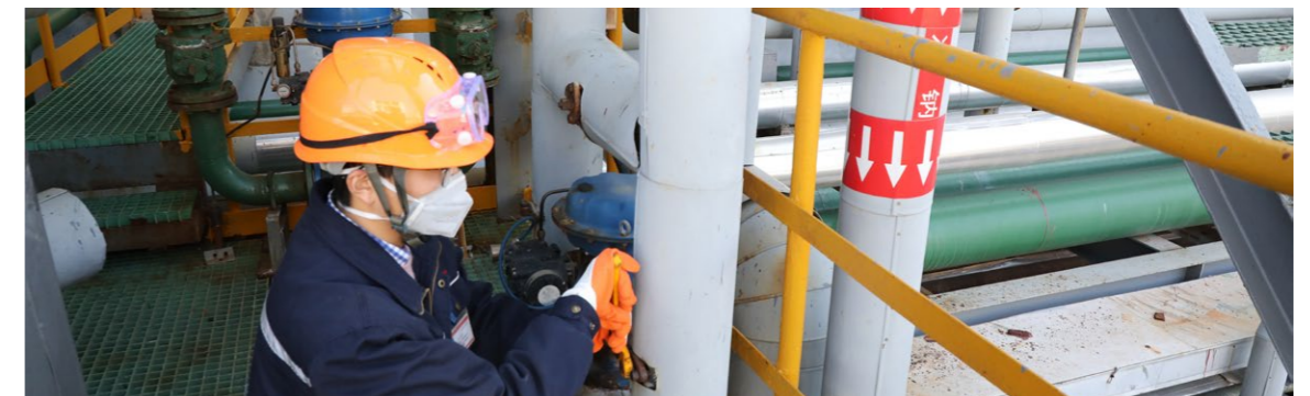
Yangnong's employees overhaul the sodium hypochlorite production facility
