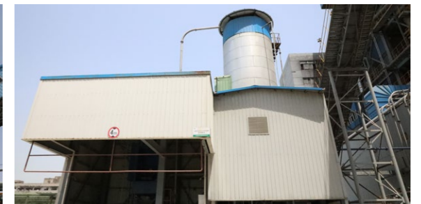
Polymer Denitrification Facility
